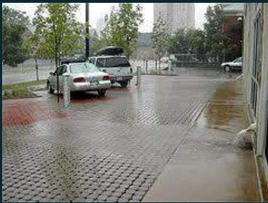
Permeable pavers reduce urban heat island effect and the demands on storm water infrastructure.
