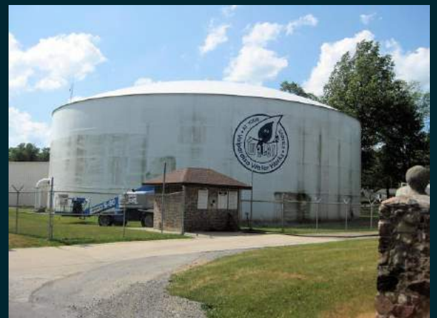
Flint Lake (North) Water Treatment Plant and Storage
