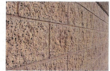
Split Face Block - Laid up in Common Bond
