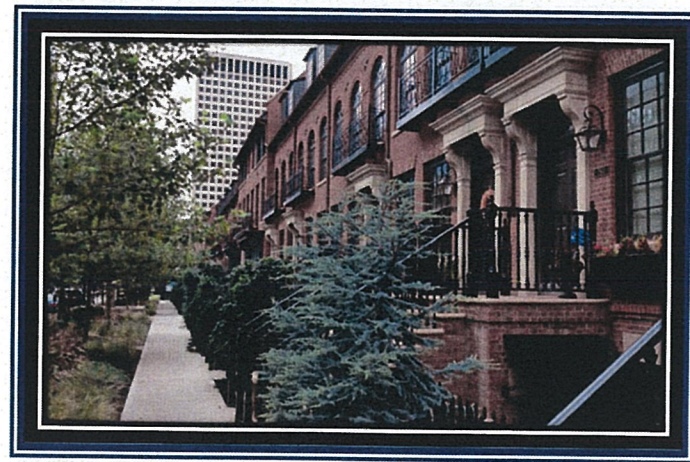
Front Façade of a "Walk-Up" building in Cincinnati We've "borrowed" many of the architectural elements, including Masonry, black windows and trim, door porticos, etc. Our "Conservation Gardens" are in lieu of the "Garden Apartments" (Basement Units)
